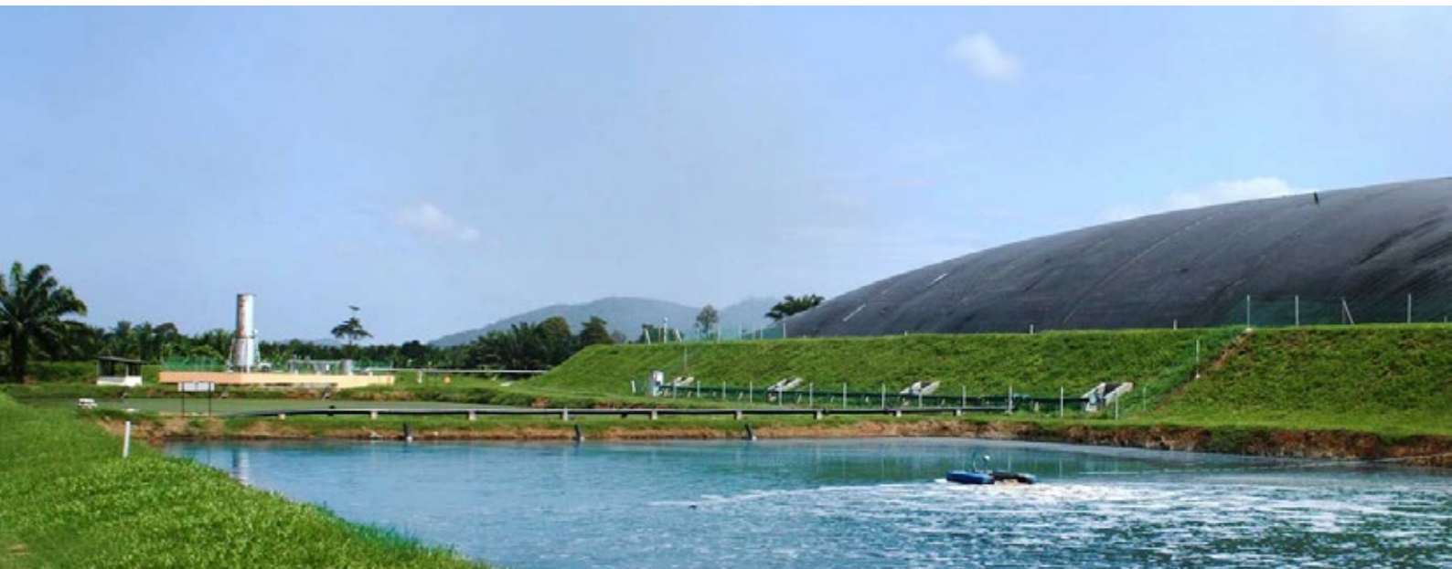
FGV's biogas power plant in Triang, Pahang. The company is continuously advancing its biogas plant initiatives and exploring alternative sources of renewable energy
